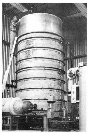
HUGE THERMOS BOTTLE — Bob Milby (8184) works on a 12-ft.-high, 2000 gal. heat storage system in Area 8. When testing is completed, tank will be moved to Albuquerque to provide heat storage in a solar energy project.
